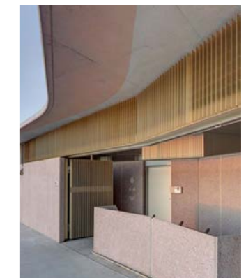
Robust material - External hand basins Mahon Pool Amenities- Lahznimmo Architects
