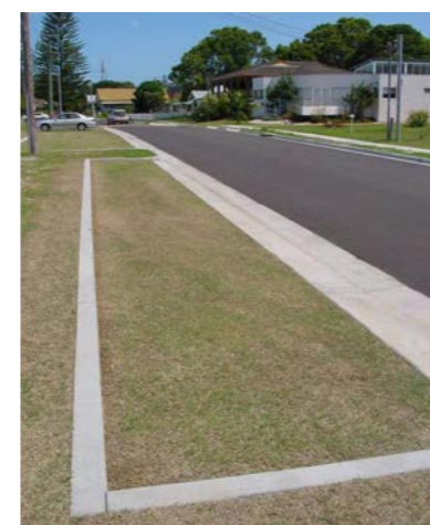
Permeable parking in marked bays
