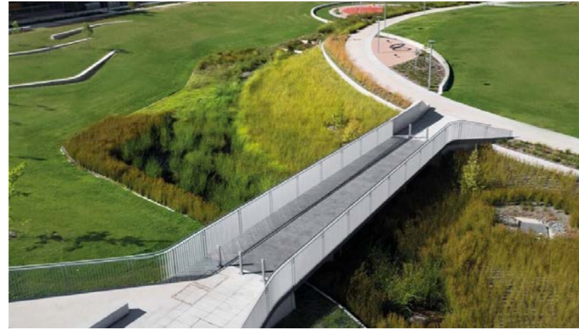
Bridge over Swales Hassett Park - JILA
