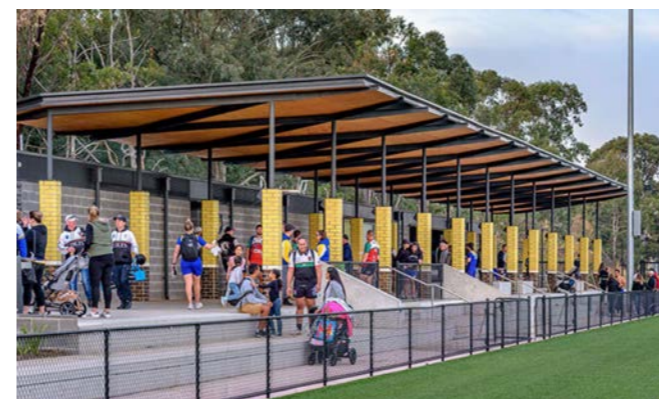
Canopy shelter and spectator bleachers NRL Amenities- Lahznimmo Architects
