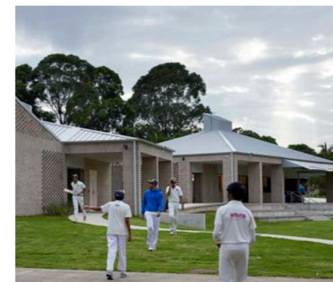
Shaded seating - Cricket Pavilion Kings Langley Cricket Club and Amenities- Eoghan Lewis Architects
