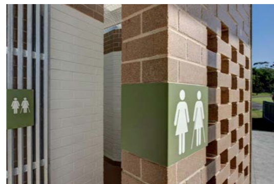
Clear and Legible signage Queens Park Sports Amenities- SCA
