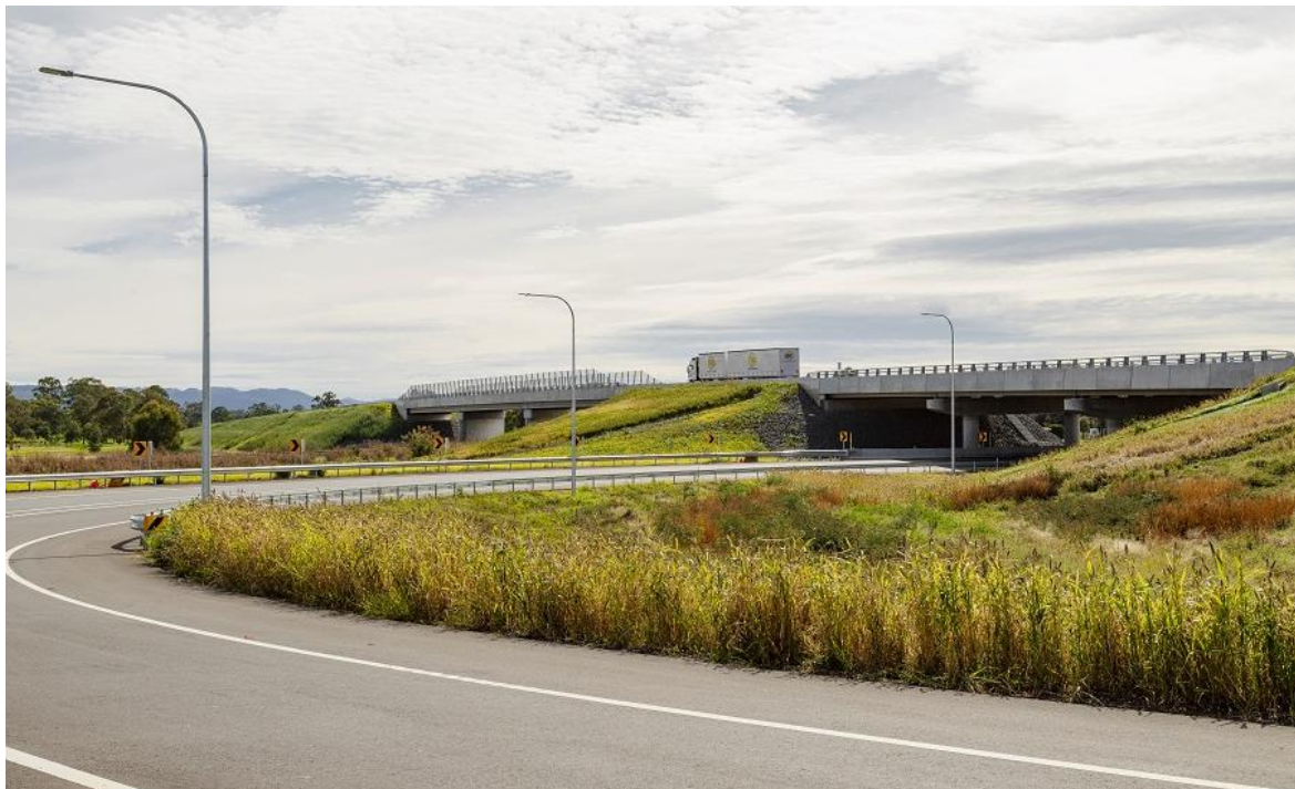
Figure 3-3 Photo of the completed Scone Bypass (source: Transport for NSW)
