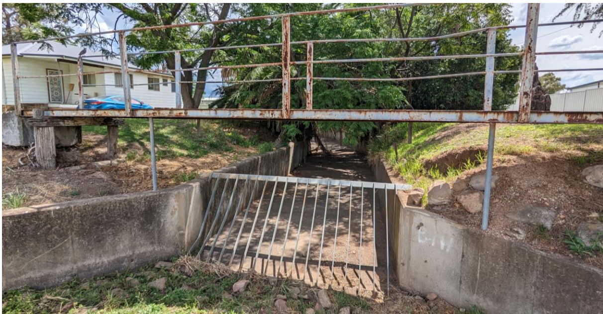
Figure 10-14 Photo of the trash rack captured in November 2023
