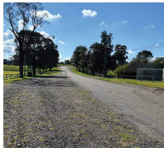
Brisbane Street dissects the two sportsground areas. Park edges are ill-defined and there are no designated pedestrian crossing points. This creates a potential safety hazard, particularly on busier days with events.
