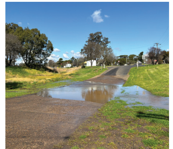
Localised flooding in Brisbane Street.
