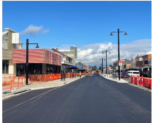
Image 3 – Intermediate asphalt Block 2 East
