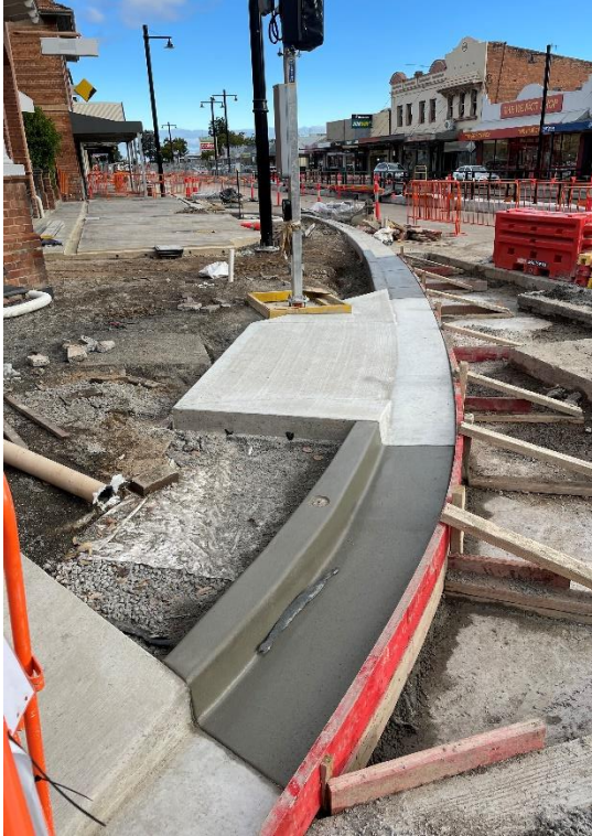
Image 6 – Kerb and Pram Ramp
