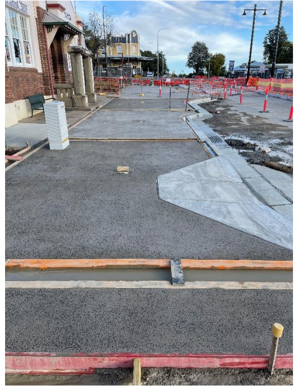
Image 7 – Footpath concrete construction
