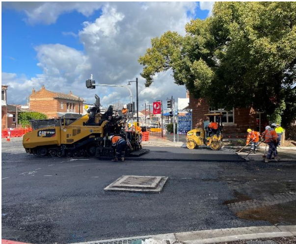
Image 2 – Intermediate asphalt Liverpool St intersection
