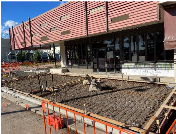
Image 3 – Footpath Form Work
