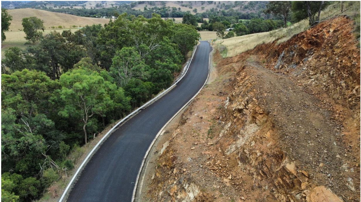
Moonan Brook Road – 1 st Cutting
