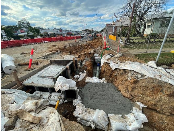
Image 6 – Stormwater Pit, Water Main
