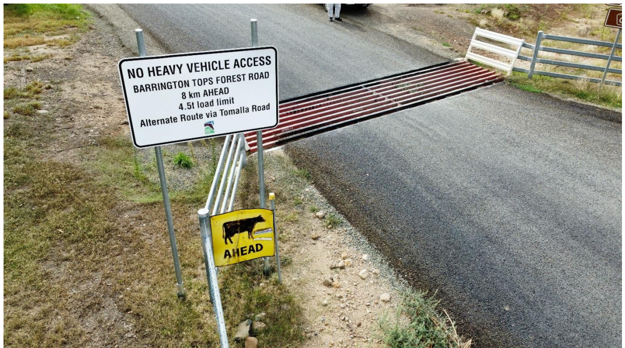
Barrington Tops Forest Road – Dual Lane Cattle Ramp at Chainage 40
