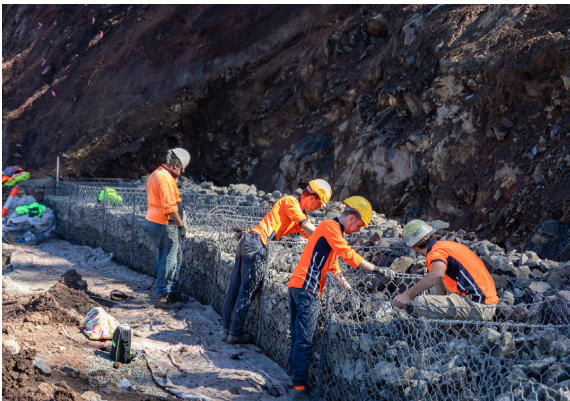
Gabion wall construction
