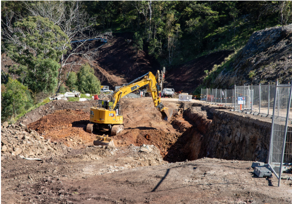
Excavations for gabion wall construction
